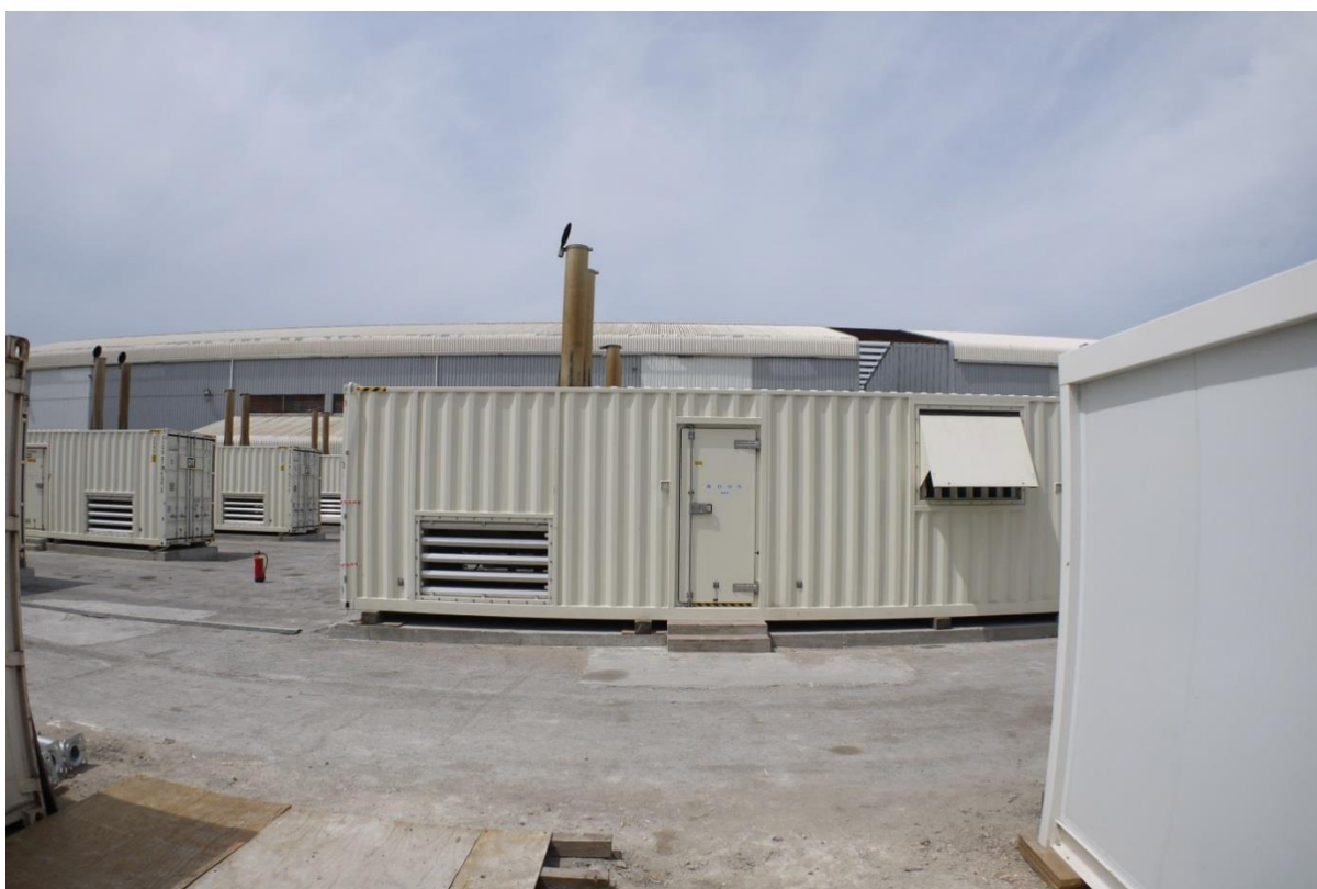
Figure 4-3: New skid-mounted generators at North Mole (2014)
